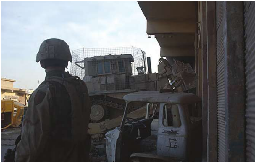
A soldier of the 82d Engineer Battalion observes as a Marine Corps D9 armored bulldozer aids in clearing a building in Fallujah. The wire cage around the cab was a defensive measure against rocket-propelled grenades.
