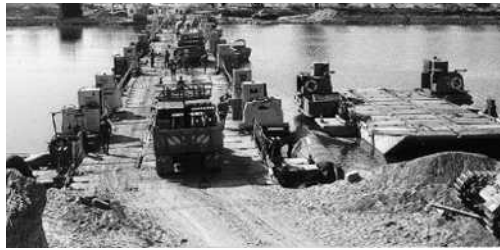
Crossing the canal on the pontoon bridge. Photograph courtesy of Israeli Government Press Office
