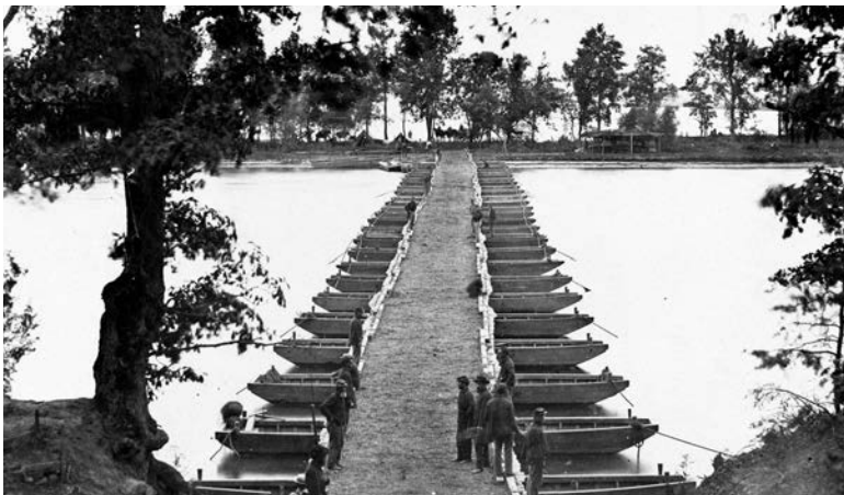
Union pontoon bridge on the James River at Deep Bottom (Library of Congress)
