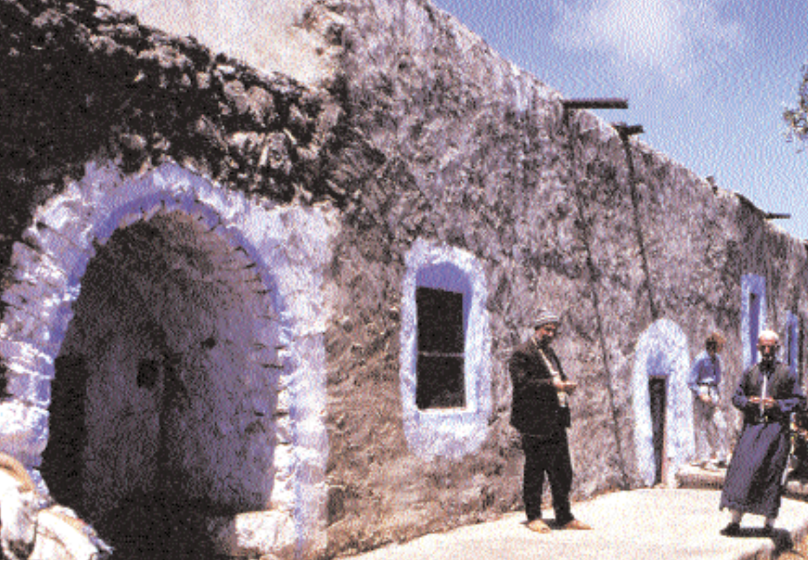
27. Building housing the tomb of Sinan near al-Kahf.
