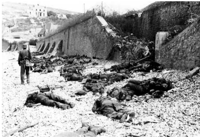
7. The aftermath at Blue Beach, called “a massacre” by John Mellor, and “a pathetic monument to poor planning and the inflexibility of the planners back in Britain.” Survivors had sheltered behind the buttresses that supported the sea wall.
