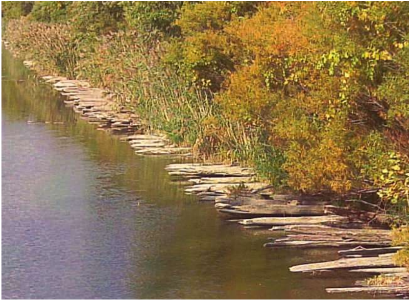
Remnants of a military corduroy road is shown near present Brownstown Charter Township, Michigan, near the mouth of the Huron River on Lake Erie. This type of road was built of logs, placed side by side, to form a traversable road over low or swampy areas. (Courtesy of author)
