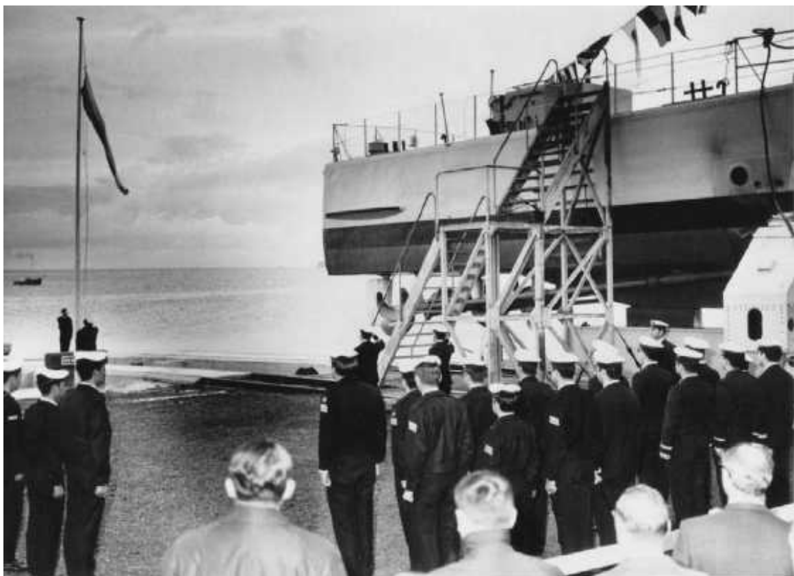
The crew of one of the missile boats standing in formation prior to a launching. At high tide the vessel would be pushed stern-first on a wooden cradle along tracks running out into the harbor, until it floated free.
