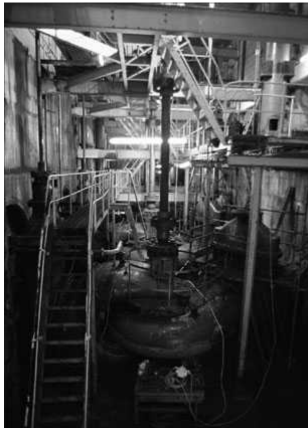
The pump room deep underground the King George V Dry Dock in Southampton. Lt Chant and his men practised over and over on these pumps, perfecting the skills needed to carry out their demolition tasks during the raid. The layout of this pump room differs from that in St Nazaire in being smaller and more confined. Note the long shafts which connect the pumps with the motors in the power room 40 feet above.
