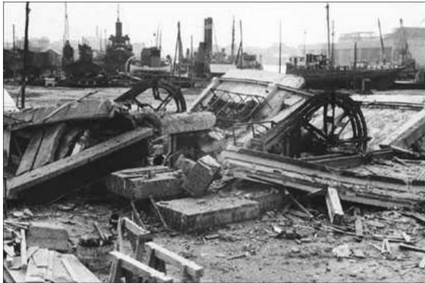
The northern winding shed after Lt Purdon and his demolition team got to work on it. The remains of the great wheels providing the momentum to draw the caisson along its camber can be clearly seen in the centre of the photograph. The background to the picture is the Submarine Basin.
