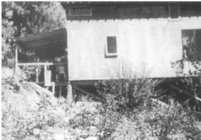
The Weaver cabin in the mountains of North Idaho in the summer of 1984, when it was completed. The cabin was built by Vicki and Randy with two-by-fours, plywood, and scraps from a nearby sawmill.
