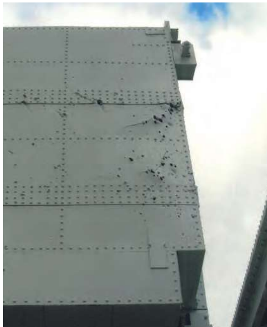
Pitting in the bridge's counterweight bears witness to the violence of the fighting that followed its capture. The 'splash' of holes and the angle of penetration suggest that this was from an exploding mortar round. (WF)
