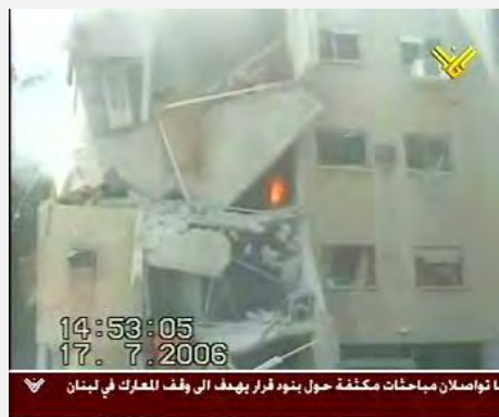
An apartment building in Haifa which collapsed after being hit by a 220mm Syrian-manufactured rocket on July 17
