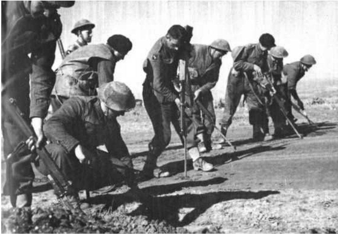
The retreating Germans mined the main Thala to Kasserine road very heavily. Members of 8th Field Squadron, Royal Engineers probe the road
